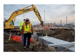
materials. This project also requires that over 1,000,000 cubic yards of fill dirt be brought onto the site to raise the ground levels on average 9' above pre-flood levels. The plan requires that this entire area be brought up level with or 2'-3' higher than the repaired levee. The site preparation portion of this project will lay out the utilities and the individual sites for the eventual construction of the various new campuses that will replace the lost facilities while at
