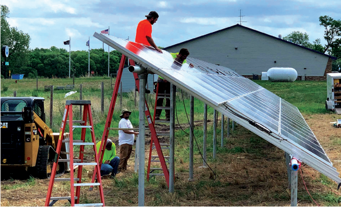
Construction of solar panel racks at Macy Campus in progress.
