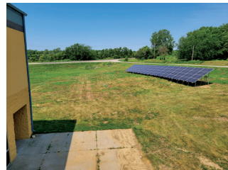
Completed panels at Macy Campus.
