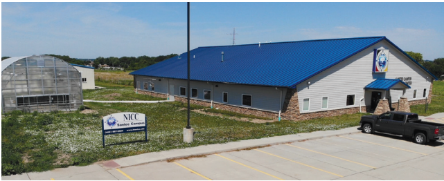
From the sky - completed connection between science lab and Santee's new aquaponics/green house facility.
