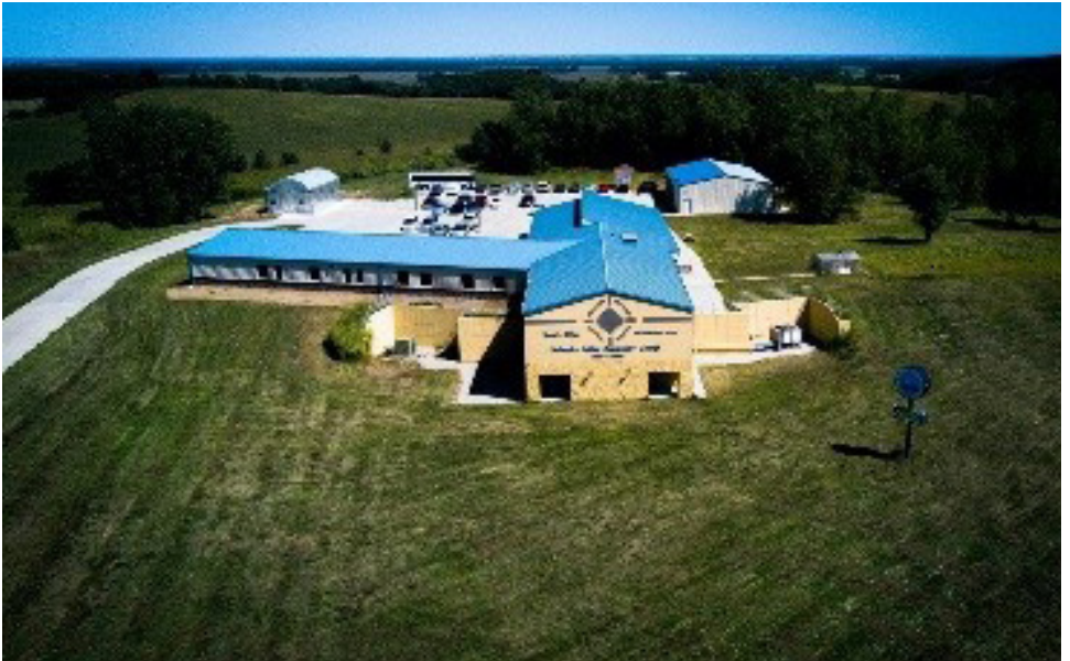
Ariel view of the Macy campus with the new wing taken in Fall of 2019.
