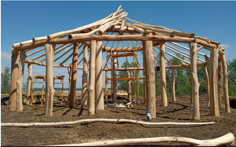
Earthlodge under construction, located on NICC's Macy Campus
