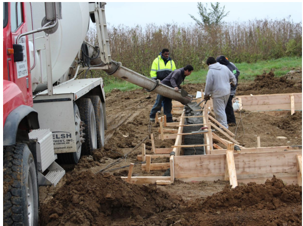
Contractors pour the footer for the aquaponics building at Macy Campus
